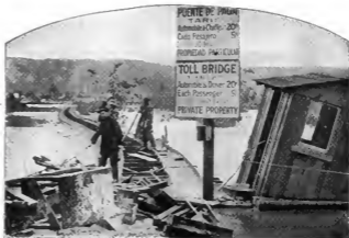
Tia Juana cut off by floods—the auto and foot bridge to the Mexican border propped and guarded to prevent its collapse during high water. (J. Bassett.)
